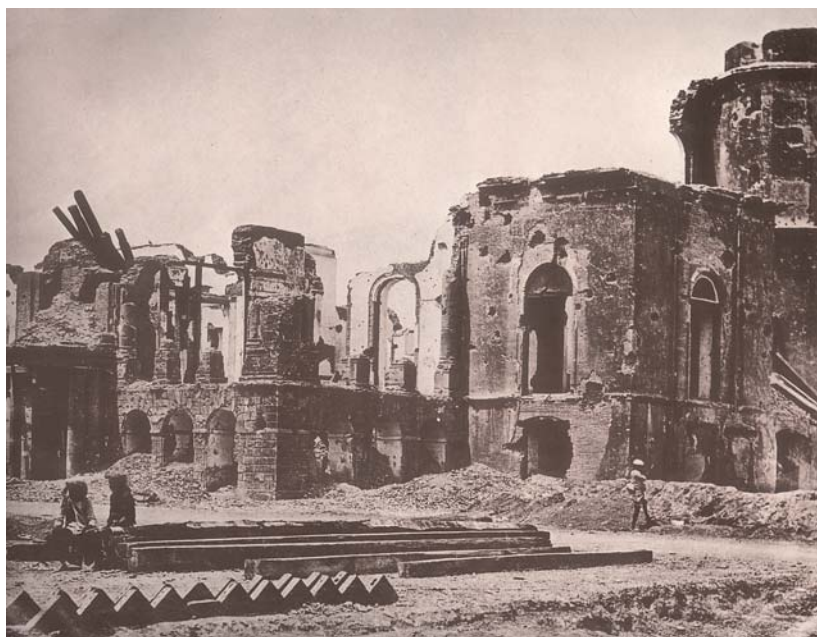
Fig. 12 – Ruins of the Residency in Lucknow
